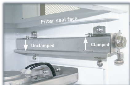
Secure and Easy Filter Change using Active Clamp System (ACS)
